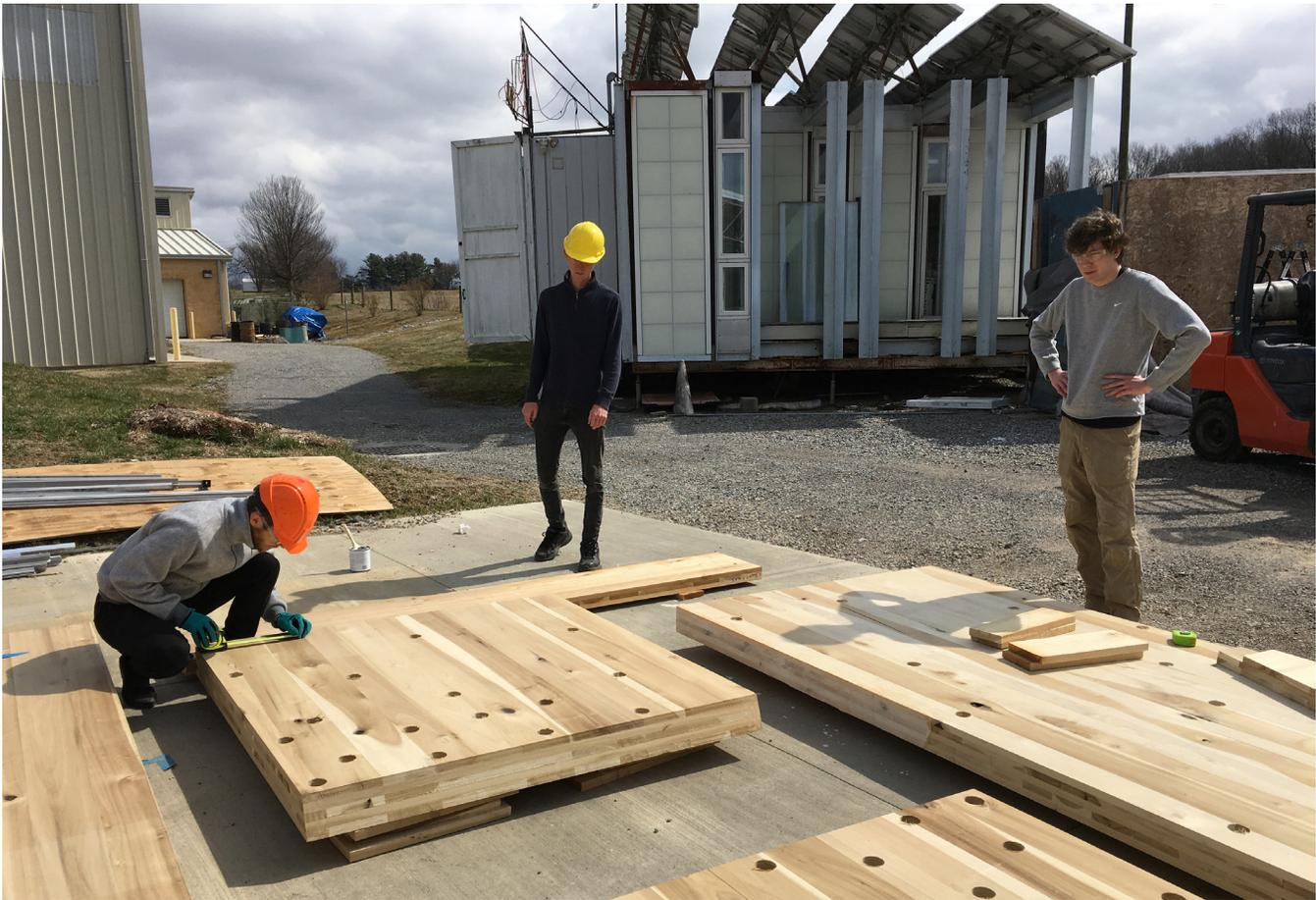
Figure 3. Custom-developed hardwood CLT from local forests before assembly.
